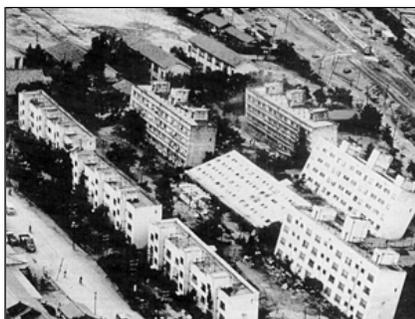
FIGURE 3 - THESE BUILDINGS IN JAPAN TOPPLED WHEN THE SOIL UNDERWENT LIQUEFACTION.
