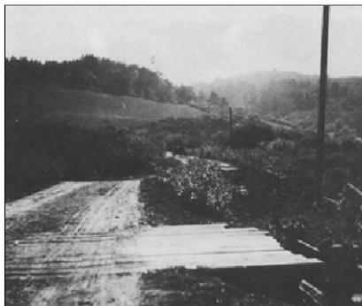
FIGURE 4 - THIS ROAD, WHICH CROSSES THE SAN ANDREAS FAULT, WAS CUT IN HALF BY THE 1906 EARTHQUAKE. ONE END OF THE ROAD SLID 20 FEET (6.5 METERS) PAST THE OTHER DURING THE QUAKE.
